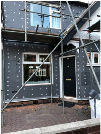
During external insulation work and after work finished.
