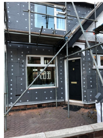
During external insulation work and after work finished.
